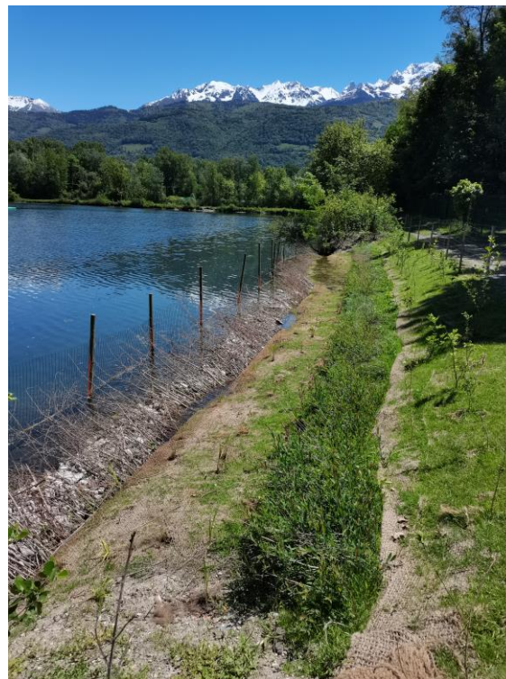
Figure 2. SWB structures using plants of different species and with a strong soil stabilization power thanks to their root development. These works help protect the bank from erosion.
