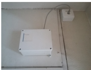
Figure 3. “EnergIST” platform: Interface with the user ( box above ); the modbus gateway receives information from the meters and sends it to the IST computer network ( box below ).
