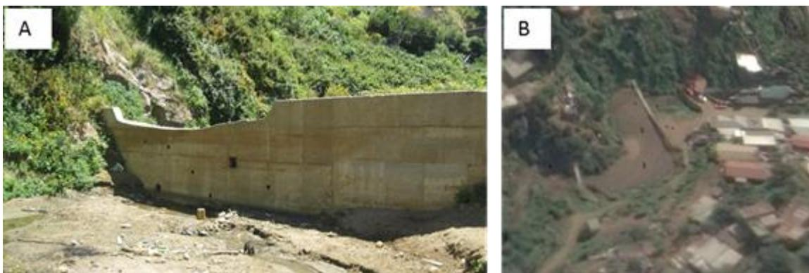
**Figure 2.** Sand trap at Francia Creek watershed exit. (A) Sand trap after clean-up of upstream side. (B) Mudflow filling up the upstream side of the sand trap after a series of heavy rain events.
