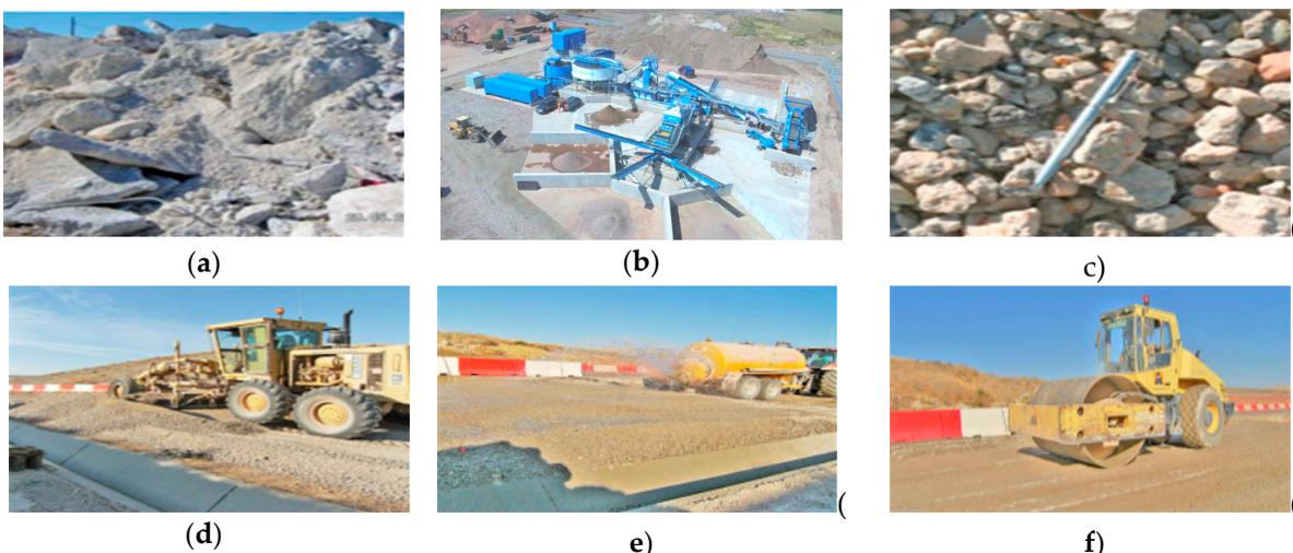
**Figure 10.** Common steps for the construction of a road pavement with CDW aggregates: (a) initial waste material; (b) Grinding and classification of various components in a fixed plant (credit: Brewster Bros); (c) CDW final product; (d) spreading and layering; (e) moisture control and (f) compaction [30,57].
