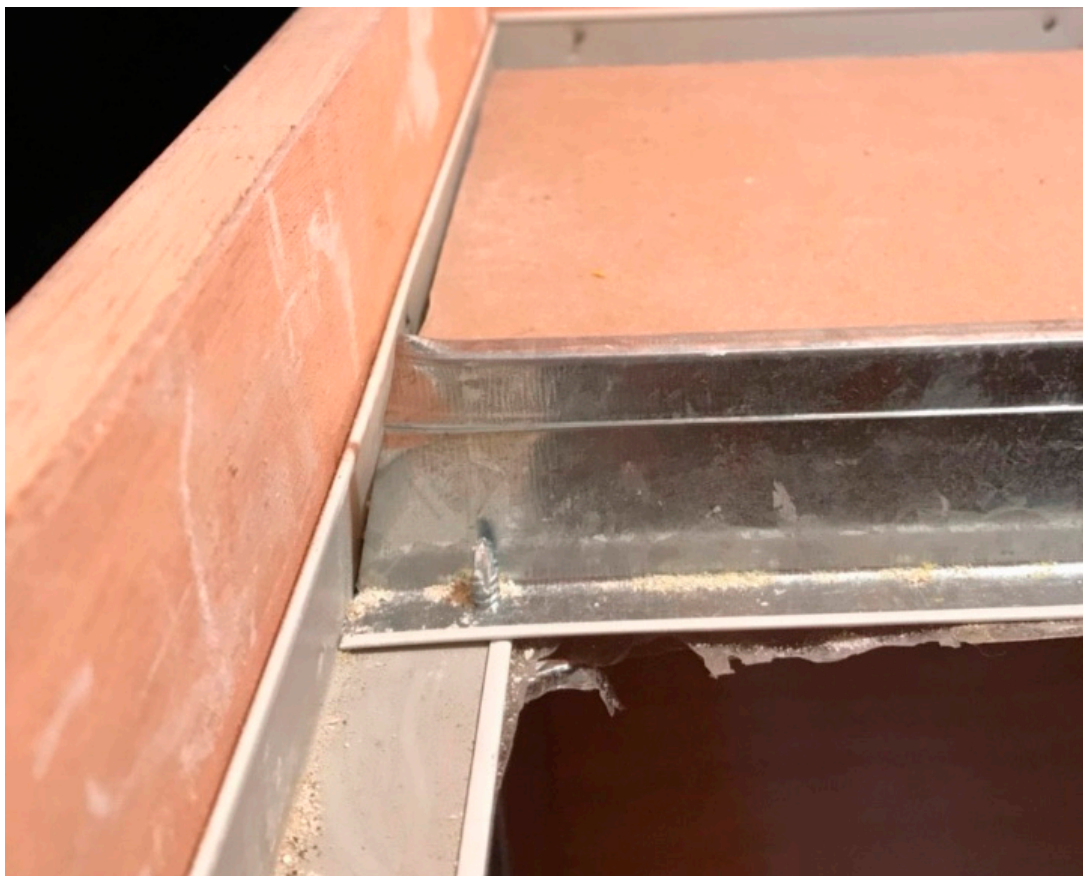
Figure 7. Junction of the grid and the trimming material after cutting.
