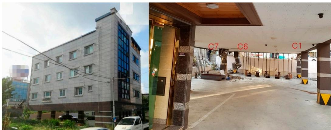
**Figure 1.** Piloti-type building before and after the earthquake event.
