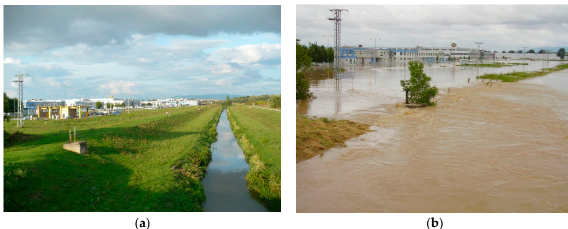
Figure 3. (a) Industrial park in Vrábľe with an average flow of water in the river Žitava (2017); (b) industrial park in Vrábľe in June 2010. The river Žitava created a new riverbed, which passed through the industrial park and poured into the main riverbed in front of the bridge (2010). (Photo: M. Izsóff).
