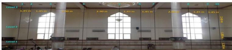
Indoor Eastern Elevation for Al-Hayyani Mosque
