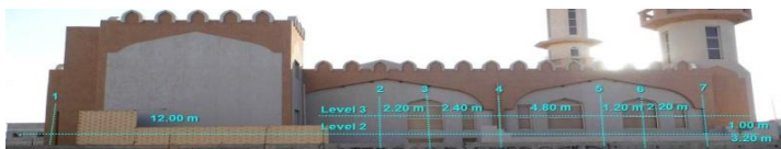
Outdoor Eastern Elevation for Noor El-Eeman Mosque
