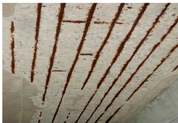
Figure 2. Concrete spalling as a result of rebar oxidation.
