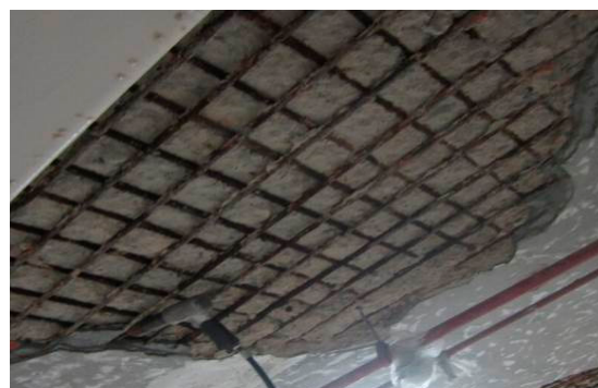
Figure 7. Coating grout crevices at the slab base with low viscosity epoxy resin.
