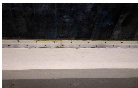
Figure 11. Affixing CFRP patches using angle steels.
