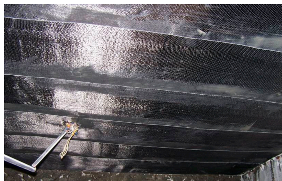
Figure 9. After CFRP patch attachment.
