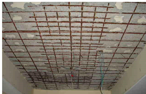
Figure 6. Concrete surface after rust removal and cleaning.
