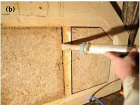
**Figure 7.** (**a**) Restoration of timber framework (**b**) TYPHABOARD infill and sealing of joints by typha swelling mortar, pictures: Fritsch Knodt Klug.
