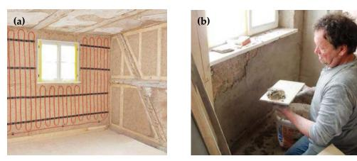
**Figure 8.** (a) Covered surface and screwing of the heating system, picture: Fritsch Knodt Klug (b) clay plastering on internal insulation, picture: Alexandra Fritsch.
