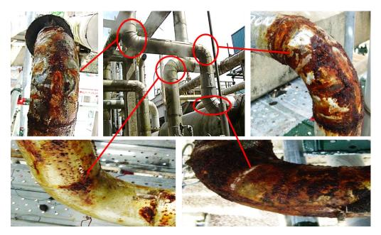
Figure 1. Corroded pipes found after the removal of insulation at some of the field inspection locations.
