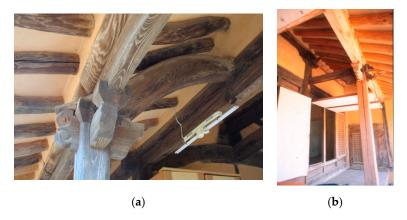
Figure 9. (a) Toetbo Beam at Unamgotaek Sarangchae in mid-Joseon; (b) Toetbo Beam at Mangcihangdan in early Joseon (source: author).
