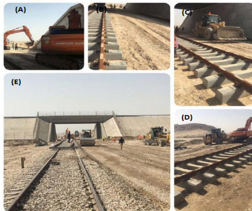
Figure 13. Images (A-D): Aspects of the repairing process for the Dammam–Riyadh train track in the study area.
