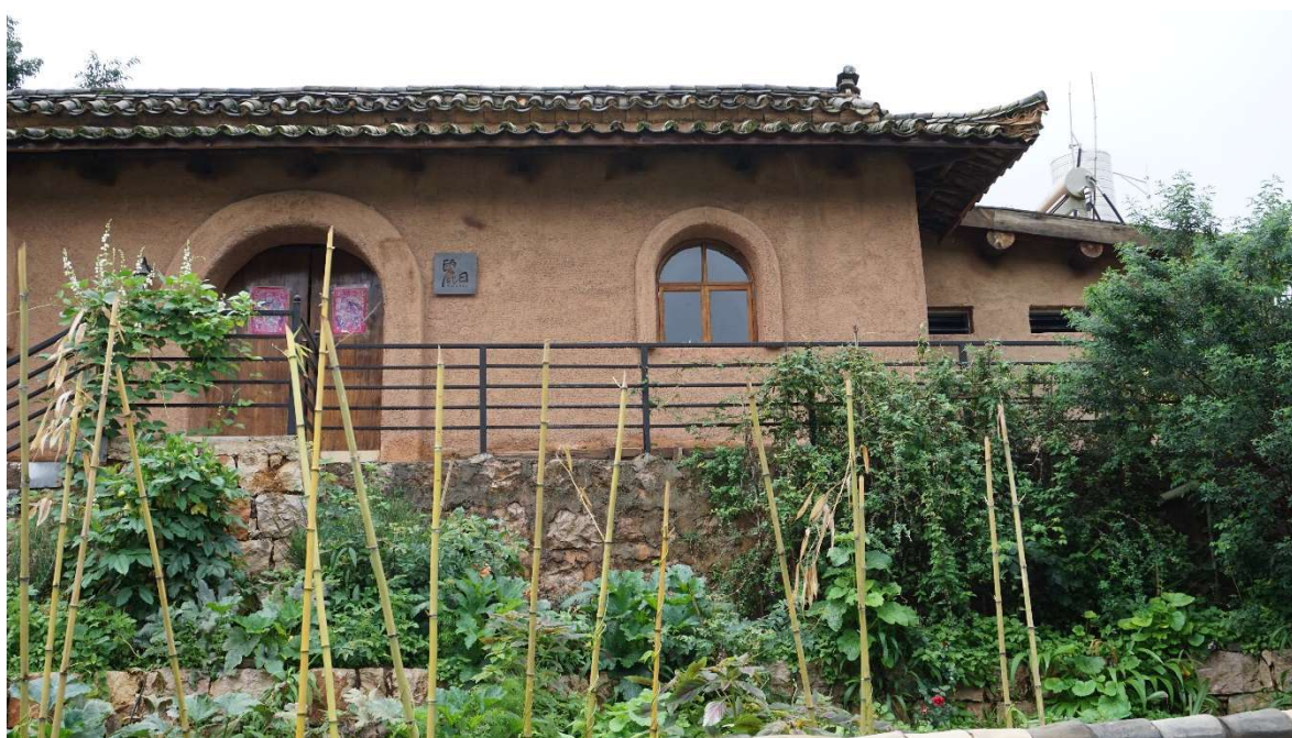
Figure 6. Damoyu—renovated mud and straw brick/adobe building.
