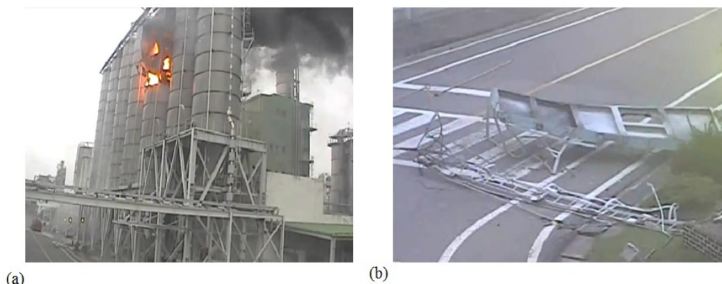
Figure 3. (a) Image of fire after silo explosion; (b) Image of upper platform deviating from silo.
