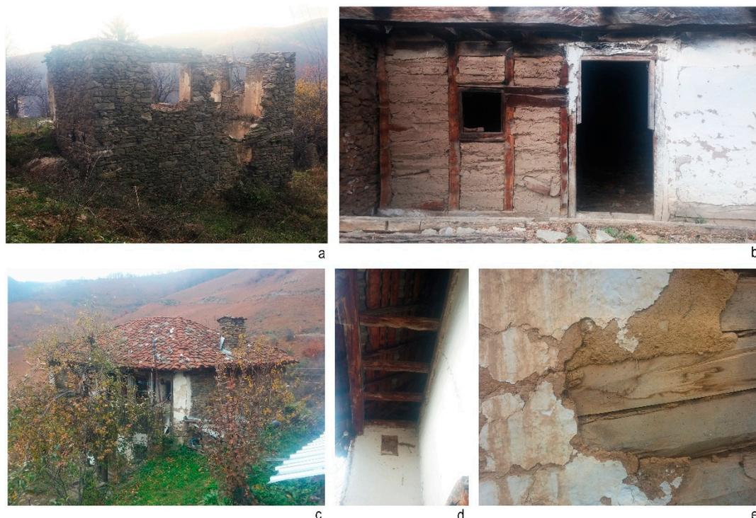
**Figure 10.** Structures and components of Sirinić houses: (a) remains of exterior stone walls of a two-story house; (b) bondruk structure; (c) original *čeramida* roof tiles; (d) roof eave structure; (e) covering of bondruk wall with a mixture of mud and straw.
