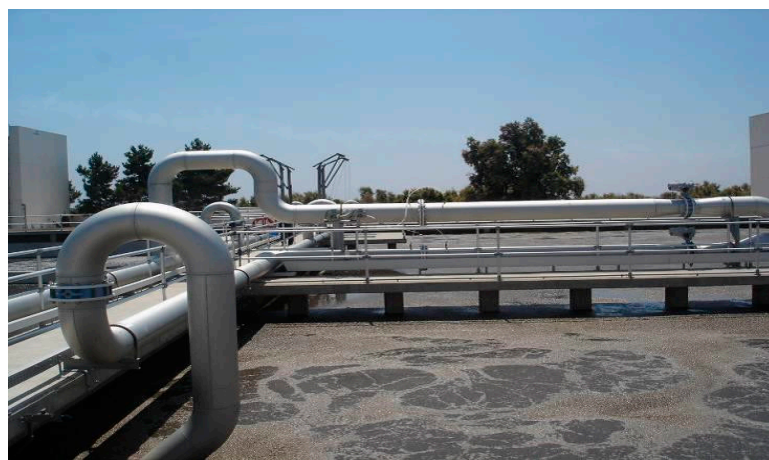
Figure 6. Biological reactor with air distribution network.
