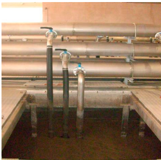
Figure 7. Membrane cassette with aeration and permeation ducts.
