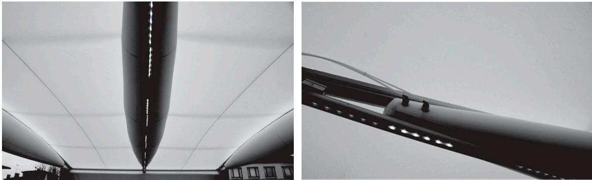
**Figure 6.** Images of the Tensairity® beam used in the Ducati Pavilion.
