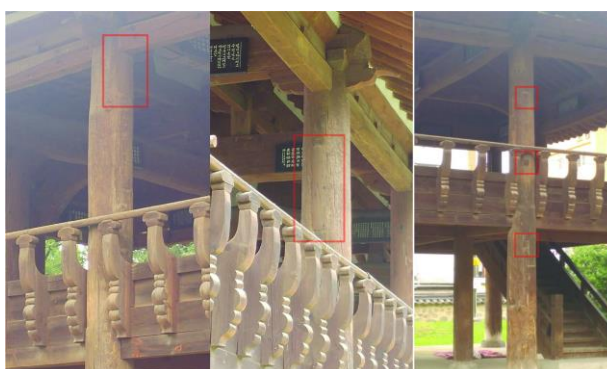
Figure 13. Traces of renovation of the exterior columns on the 2nd floor. (all figures source: author).
