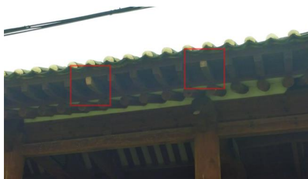
Figure 15. Traces of the reuse of wood elements. (source: author).
