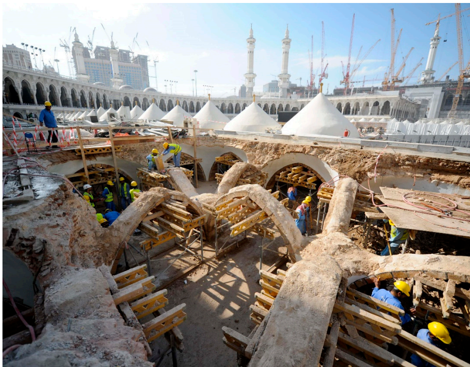
Figure 8. Dismantling and protection procedures for the archaeological arches for more sustainability.
