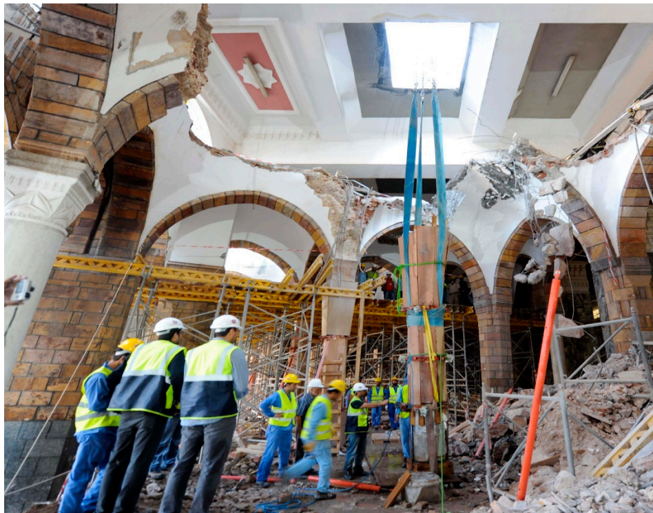
Figure 9. Dismantling and protection procedures for the archaeological columns for more sustainability.
