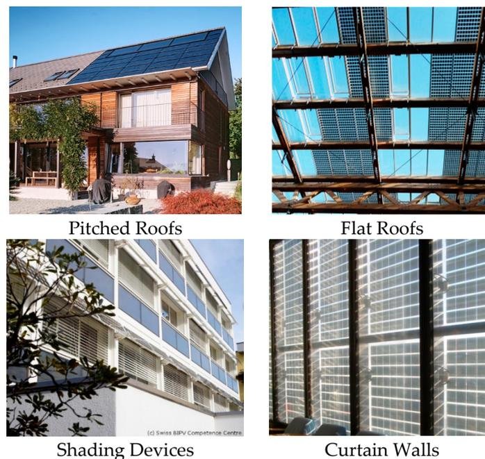
**Figure 1.** Some integration forms of photovoltaics into building facades [15].
