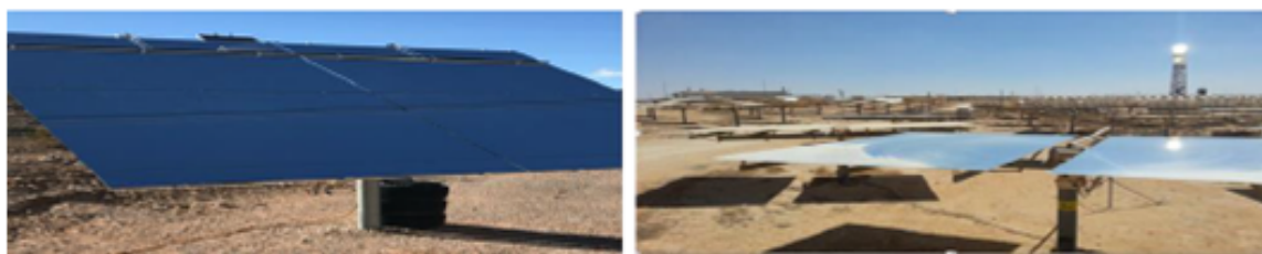
Figure 5. Images of 1st (right) and 2nd (left) generation integral cleaning devices installed on a heliostat in BrightSource Solar Energy Development Center (SEDC).
