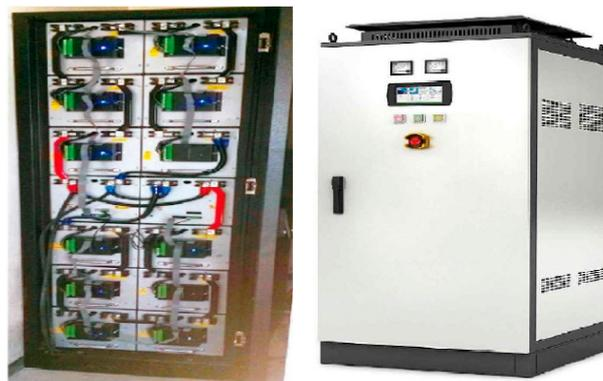
Figure 3. Battery (left) and PCS (right) on rooftop.
