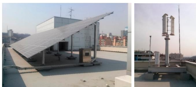
**Figure 2.** PV and WT system at the Guri office.
