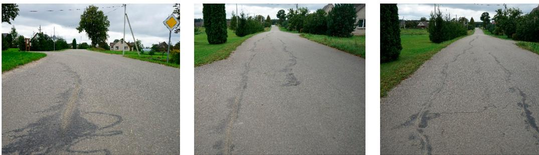
Figure 4. Sealed longitudinal cracks on road No. 2430 in summer 2017.
