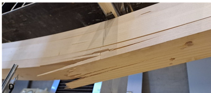
Figure 6. Characteristic failure of beam specimen with mechanically inserted dowels installed alternately through the lamellae (A), welded dowels installed alternately through the lamellae (B), mechanically inserted dowels installed vertically through the all lamellae (C), and mechanically inserted dowels with dowels installed at a 45° angle through the all lamellae (D).
