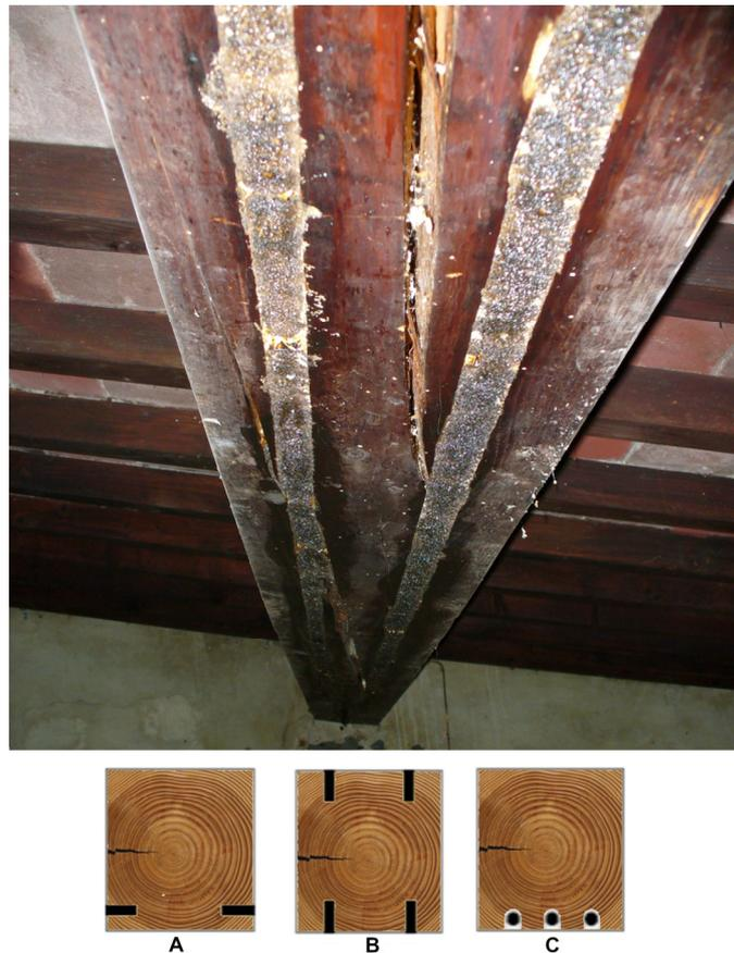
**Figure 1.** (Top): Ancient structures with an old timber beam strengthened at the intrados face via inserting steel plates into grooves routed along the longitudinal axis. (Below): Examples of some types of grooving that involve insertion for internal glued reinforcement arrangement: **A**, placing fiber-reinforced polymer (FRP) strips close to the intrados; **B**, incorporation of steel plates; and **C**, inclusion of pultruded fiberglass rods on intrados.
