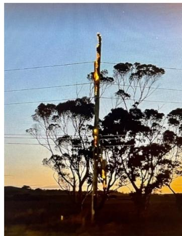
**Figure 5.** Burning pole—initiation of fire within the pole due to leakage of current or electrical apparatus fault.
