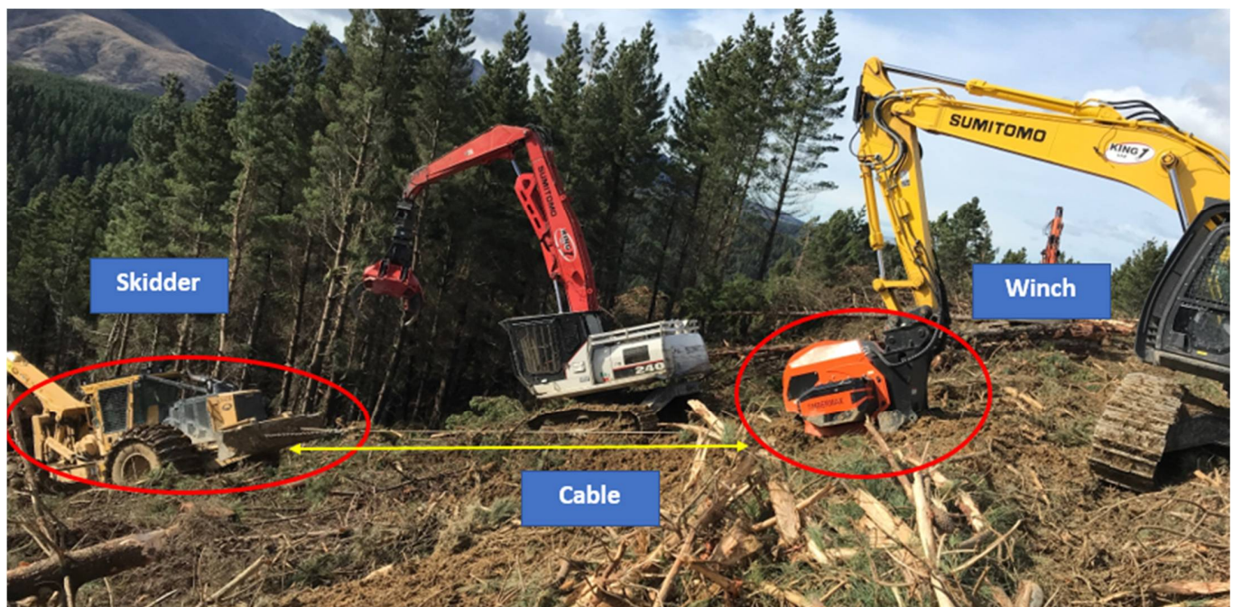
Figure 1. The Tigercat Grapple Skidder climbing towards the landing (left), the TimberMax winch on the edge of the landing (right) and the cable connecting them. The tracked loader in the centre is moving downslope to prepare the loads for the skidder.
