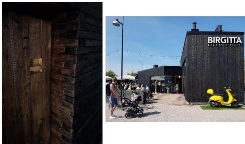
**Figure 4.** A detail of a sauna made from surface charred elements in Espoo, Finland; a restaurant in Helsinki with a flame charred exterior.
