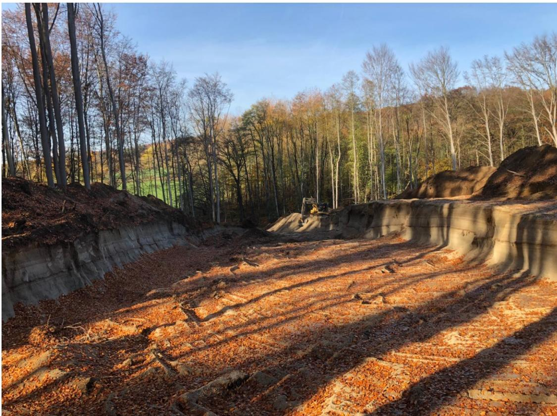
**Figure 3.** Beginning pumice excavation in forest district Bendorf, area CUT/CUT EX in late 2018 (Photo: Alexander Klein). Material for later backfilling and LST are visible on both sides. Area FOR is located on the left (West), excavation continued gradually to the right (East).
