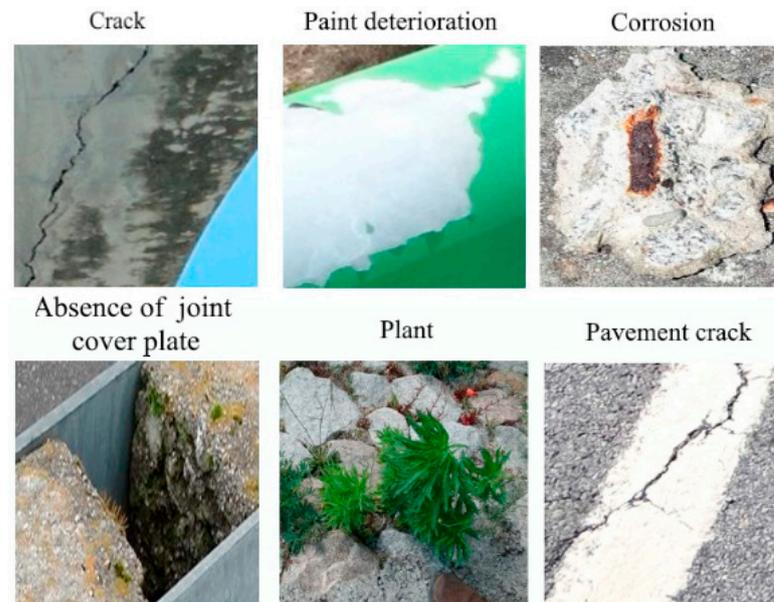
**Figure 2.** Different types of defects commonly found in bridges, which are also documented in previous work [1].
