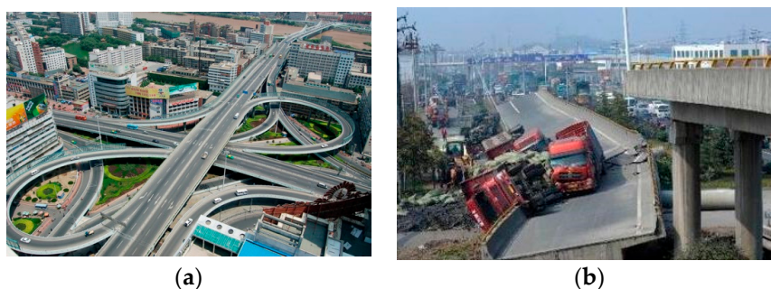
Figure 1. Perspective view and collapse of irregularly-shaped bridges. (a) Xiao Xihu overpass in Lanzhou; (b) collapsed overpass in Zhejiang [3].
