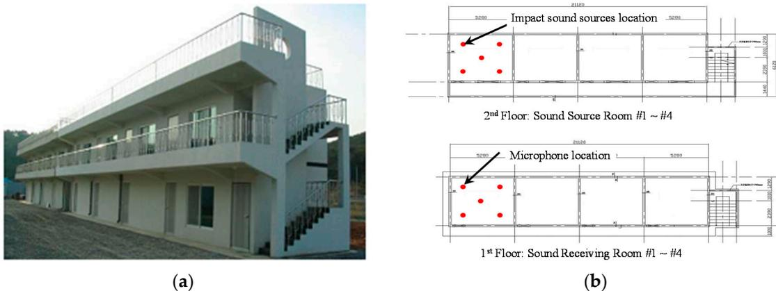
Figure 13. Overview and floor plan of the test building: (a) ISO view of the test building; and (b) floor plan of the test building.
