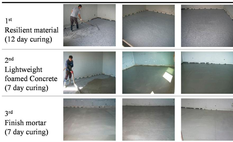
Figure 12. Construction process for floor system using resilient materials.
