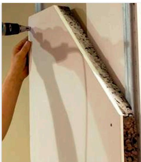
**Figure 2.** ICB glued to gypsum plasterboard in an Internal TICS (ITICS) [10].
