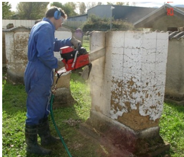
Figure 8. Cutting a wall with chainsaw.
