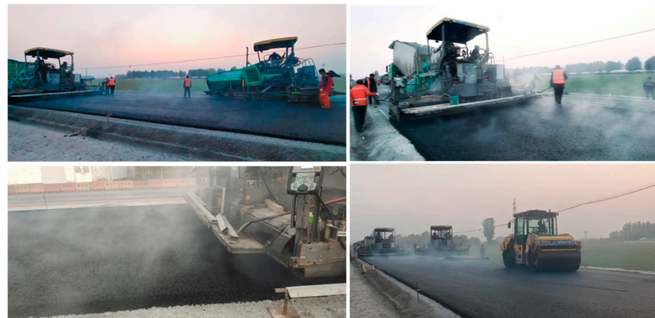
Figure 17. Laying and rolling of high-ratio DCLR-modified asphalt mixture.
