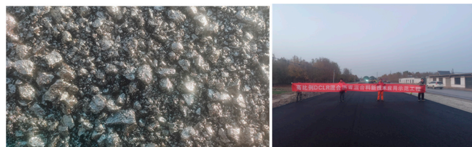
Figure 18. High-proportion DCLR-modified asphalt mixture pavement.
