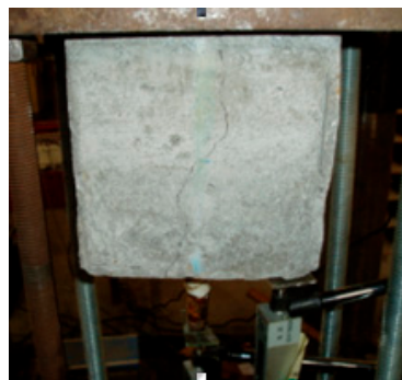
(a) Splitting failure along reinforcement
