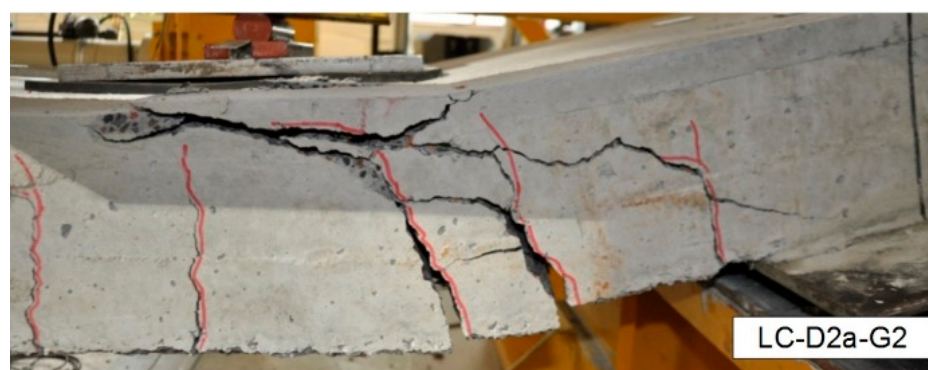
Figure 1. Typical shear failure mode of tested specimens [22].
