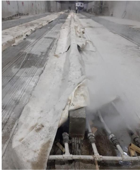
**Figure 3.** Curing of specimens via the steam method.
