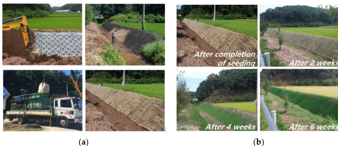
Figure 9. Slope application of vegetation porous concrete: (a) repair process [83]; (b) construction application effect [83].
