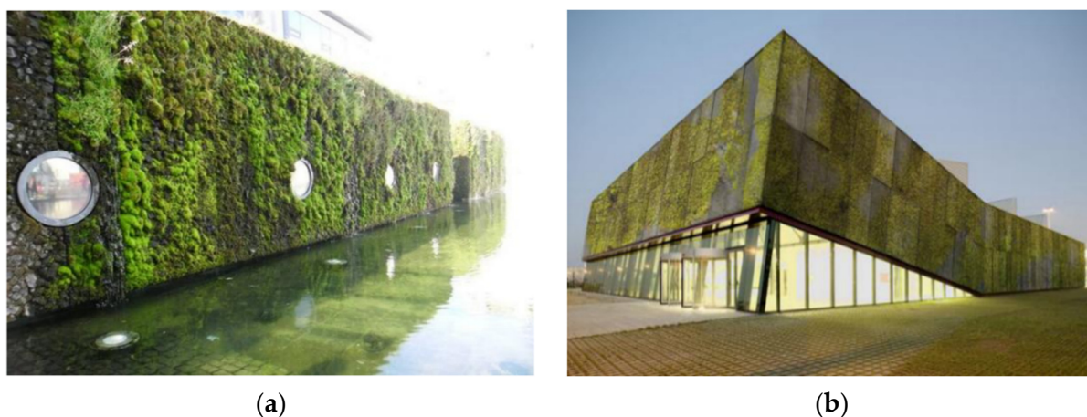
Figure 10. (a) The moss wall of the Reykjavik City Hall [9]; (b) concept of vegetation porous concrete office building construction [9].
