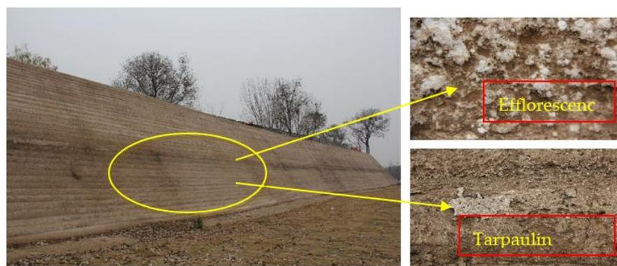
**Figure 1.** Deterioration of the Kaifeng City Wall.
