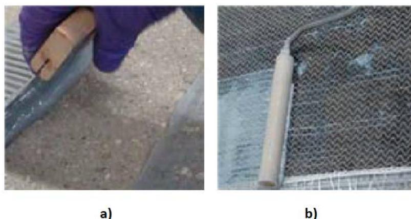
**Figure 7.** Stages in the dry lay-up process: (a) reinforcing the concrete substrate and (b) applying the FRP reinforcement to the concrete substrate, adapted from [27].
