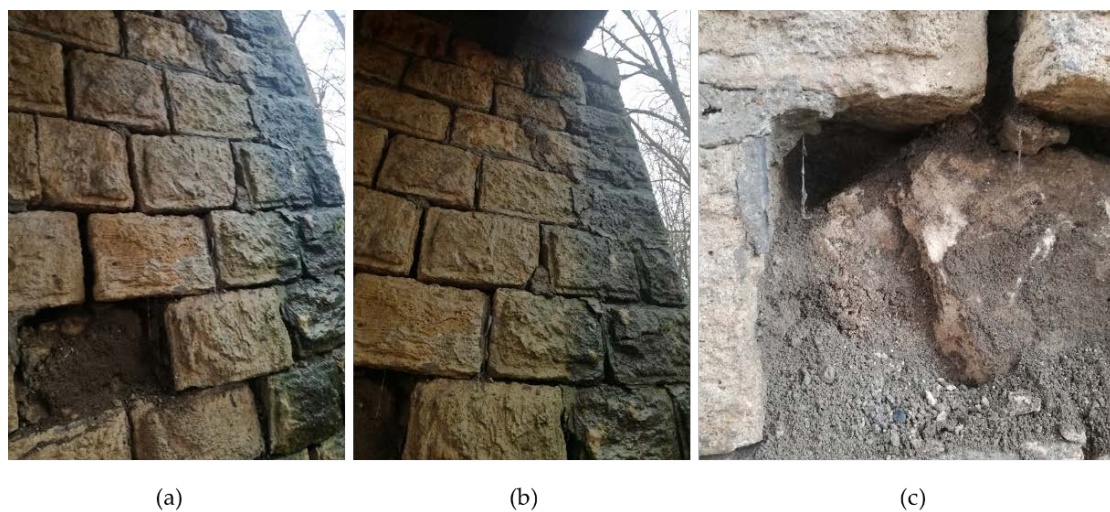
Figure 14. (a,b) Damage to the masonry walls of the abutment; (c) escarpment of infill material from the abutment.
