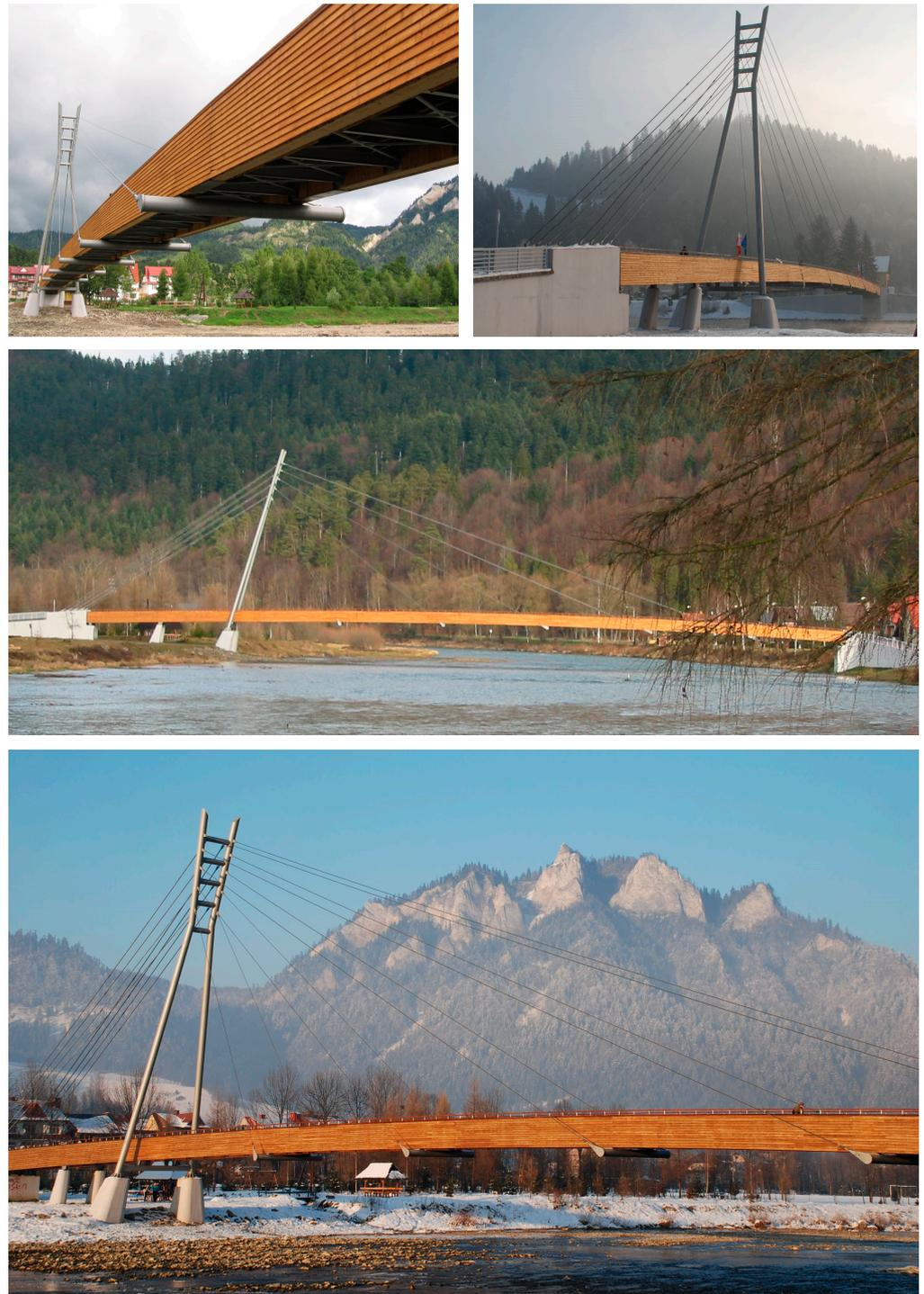
**Figure 2.** The cable-stayed footbridge in the Pieniny mountains made of glued-laminated wood.
