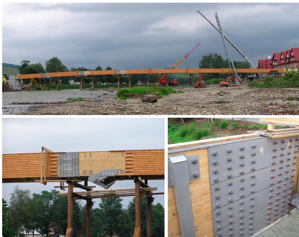
**Figure 12.** Installation of the deck on the temporary supports and assembling joints in the wooden girders.
