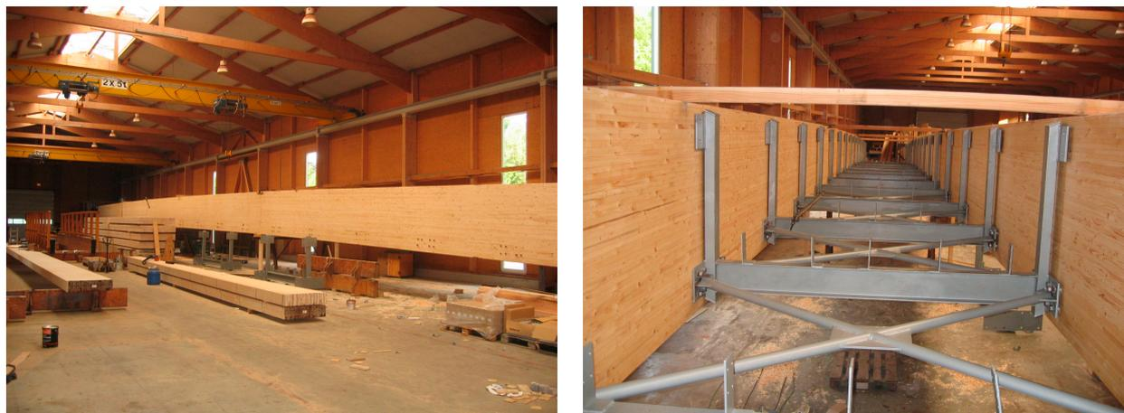
**Figure 1.** Environmental-friendly glued-laminated wood used for construction of the footbridge's main girders and the deck (Photo credit: Schmees & Lühn Holz- und Stahlingenieurbau GmbH & Co. KG and Mosty-Wroclaw Design & Research Office).
