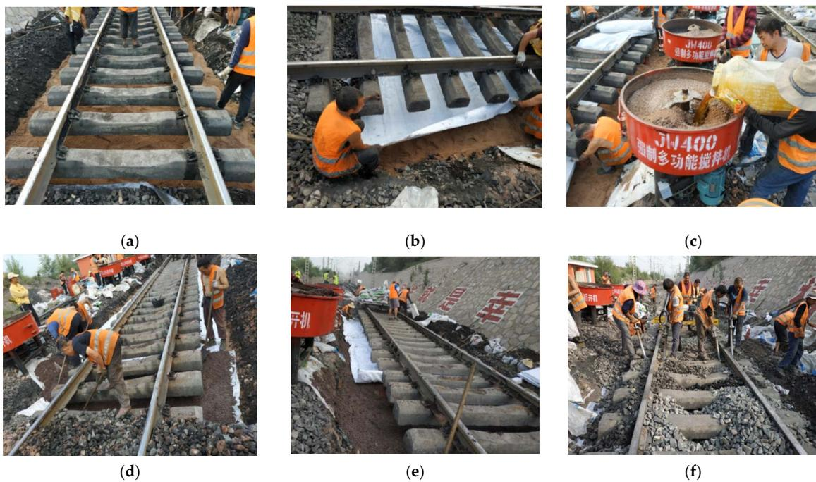
Figure 8. Structural drawing of the waterproof PP-improved gravel layer: (a) laying sand cushion, (b) laying bottom geotextile, (c) Mixing of PA, (d) paving PU-GA layer, (e) laying upper geotextile and (f) backfilling and tamping ballast.
