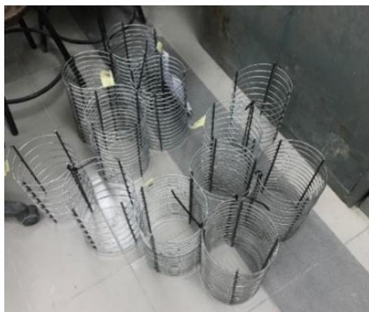
**Figure 2.** Confining hoop reinforcements.
