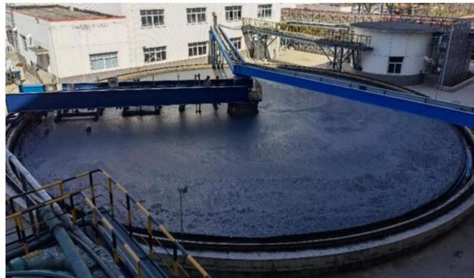
Figure 4. Layout of the thickener.
