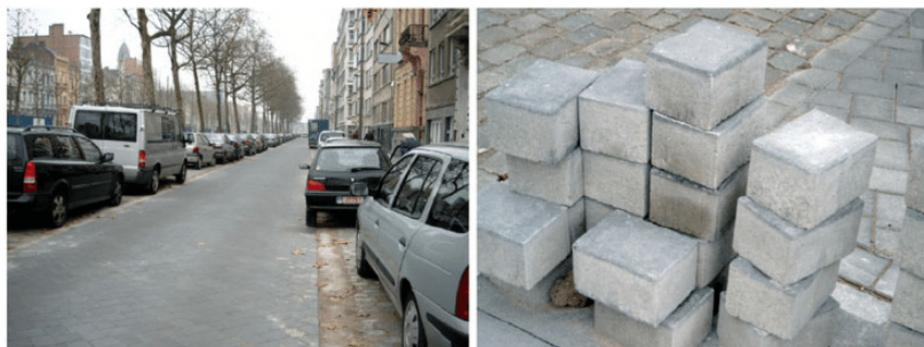
**Figure 6.** View of a parking lane with a photocatalytic paving stone in Antwerp [165].
