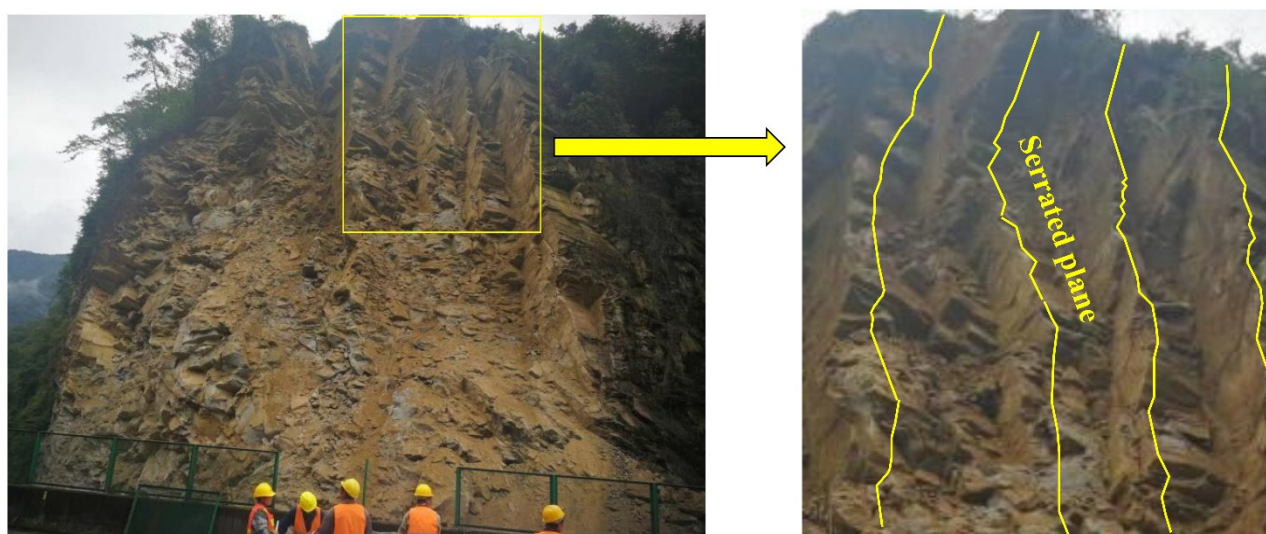
Figure 1. The distribution of one serrated structural plane of a slope.
