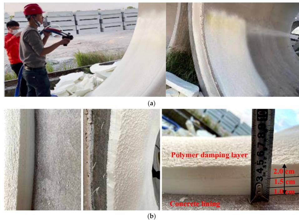
**Figure 12.** Spraying construction process of polymer damping layer and illustration of layered spraying effects: (a) spraying construction process; (b) spraying effects.
